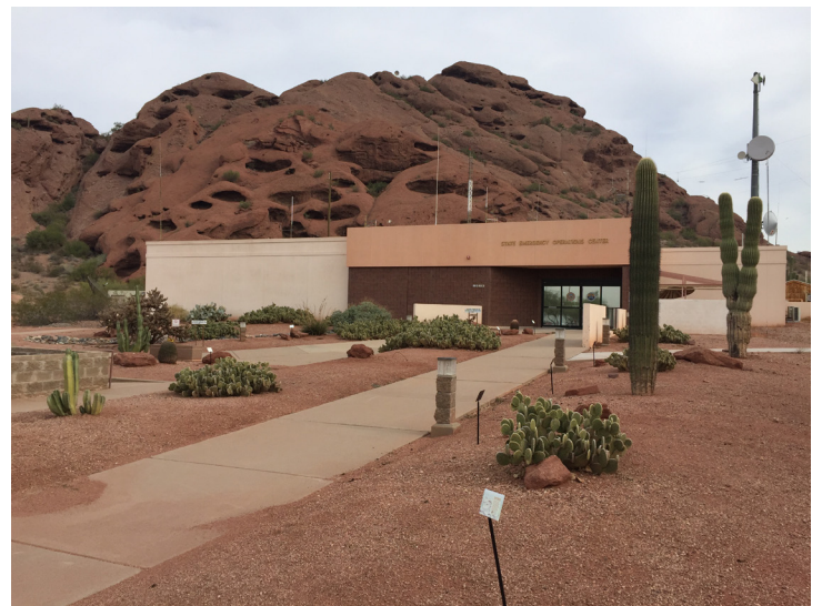
ABOVE: The current State Emergency Operations Center, built in 1983 by the Palo Verde Nuclear Generating Station as the off-site Emergency Operations Center, is undersized to manage state emergencies.
