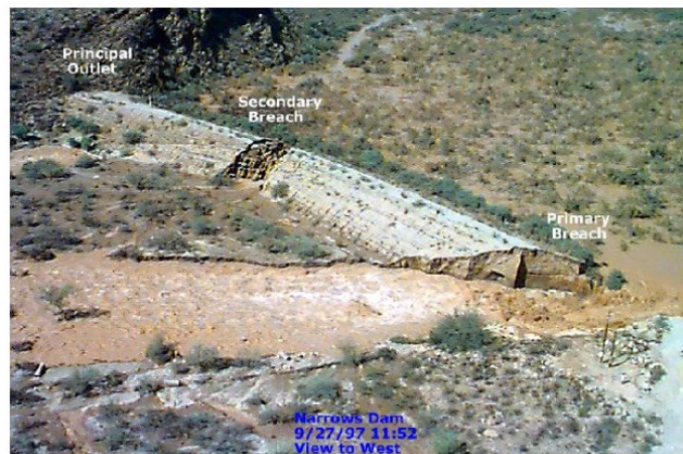
Narrows Dam – approximately 14-hours after breach failure. Source: Flood Control District of Maricopa County, 1997
