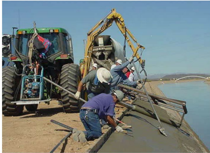
CAP Canal lining raise in Pool 24 Source: Central Arizona Project
