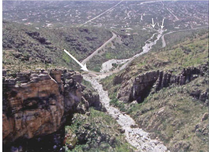
Soldier Canyon debris flow. Small arrows at top of photo show where cobbles and boulders were deposited just upstream of several homes during 2006 event (Figure 9 in reference). Source: Pearthree and Youberg, 2006
